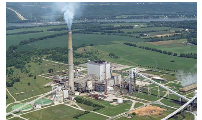
▶ East Bend Station - Ohio
