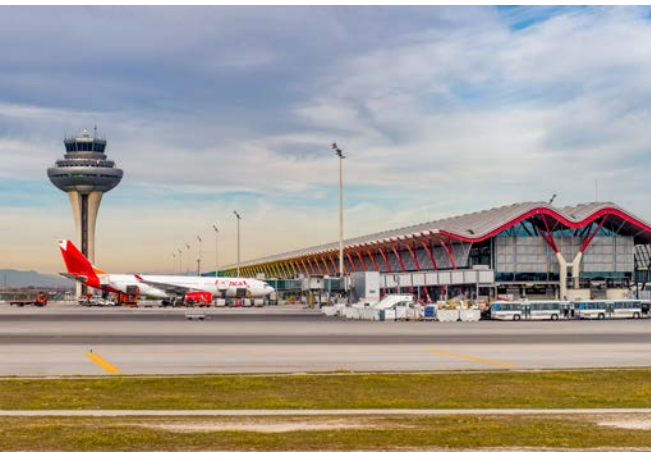
▶ Madrid - Barajas Airport
