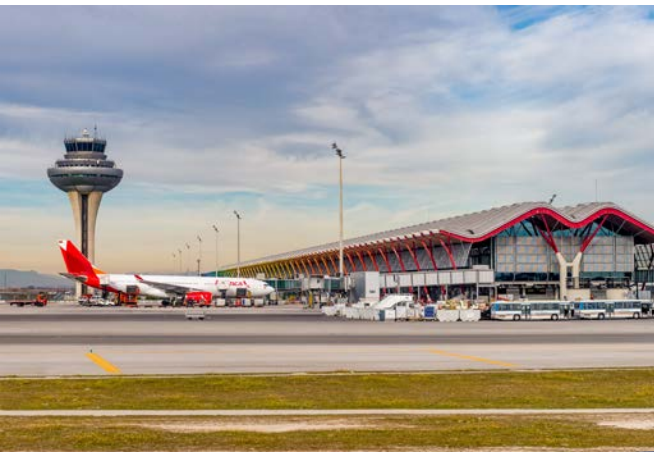
▶ Madrid - Barajas Airport
